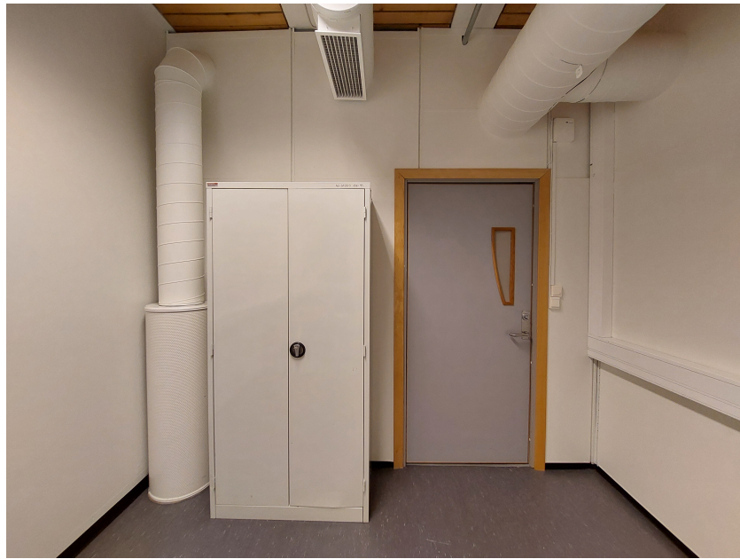
Figure 4.1: The entrance seen from inside the room.
