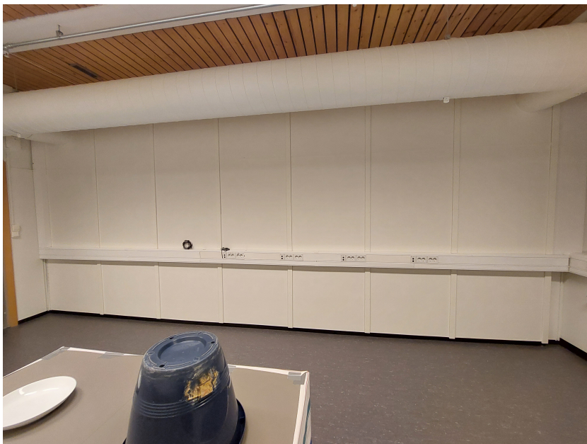
Figure 4.4: The room seen from the right wall.
