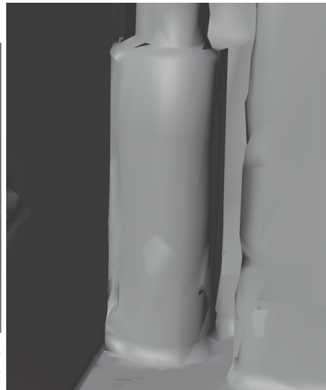
(d) Some parts of the vertical ventilation pipe have merged into the wall (4cm threshold).
