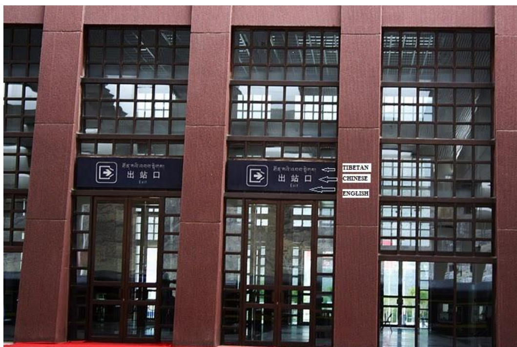
(Lhasa Railway Station, Photo: Shen Zhang)
