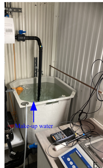
Appendix 1 Overview of the different sampling points from Sunndalsøra RAS. A: fish tank, B: outlet from drum filter, C: outlet from biofilter, D: sludge & E: make-up water.
