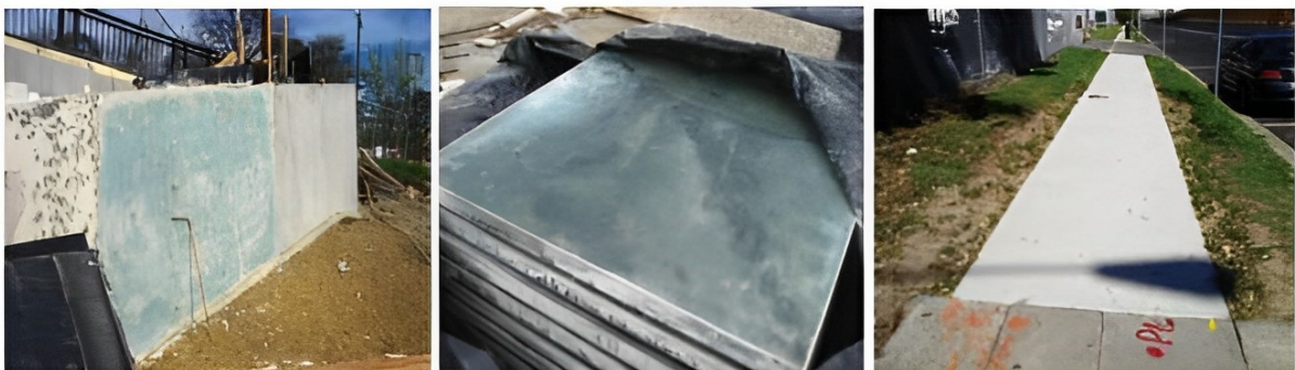
Figure 2.3: Geopolymer concrete, retaining wall (left), footway pannels (center) and footpath (right) [4]
