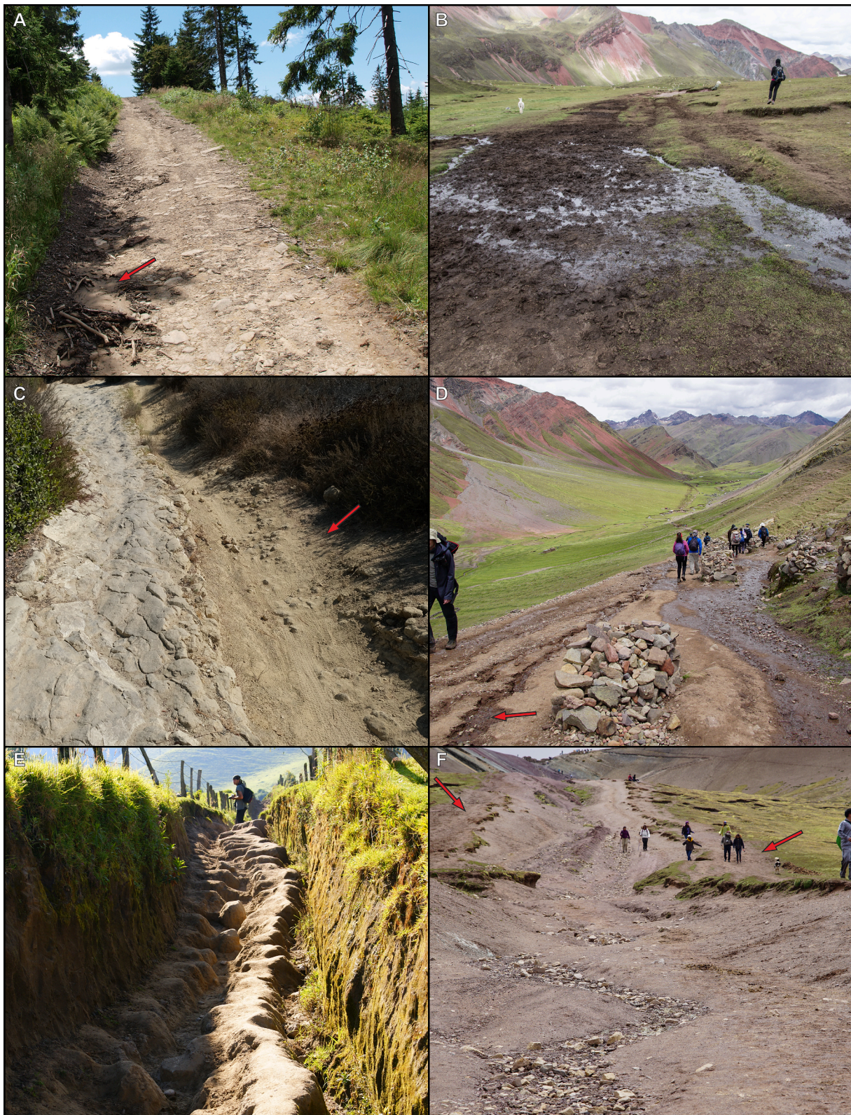
Fig. 1. Examples of trail impact: A – deposition of material (indicated by arrow) due to improper trail drainage; B – muddy section and water puddle; C – exposed bedrock on the too-narrow section of the trail, which forced visitors to trample trail sides; D – erosional rill (indicated by arrow) along the trail tread; E – deep gully reaching bedrock; F – strong trail incision and development of rills; due to uncomfortable and dangerous walking conditions, visitors created informal paths (marked by arrows) next to the designated trail.
