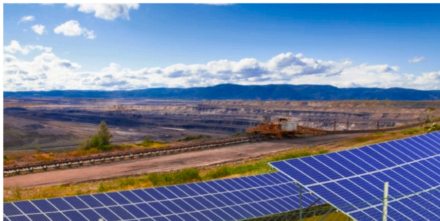
Fig. 3. Solar installation at Fekola gold mine in Mali ('b2gold.com' 2023).
