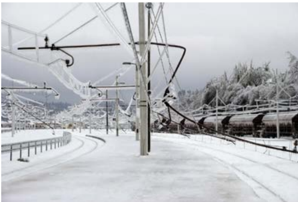
Figure 1: Example of icing on railway overhead lines [18].
