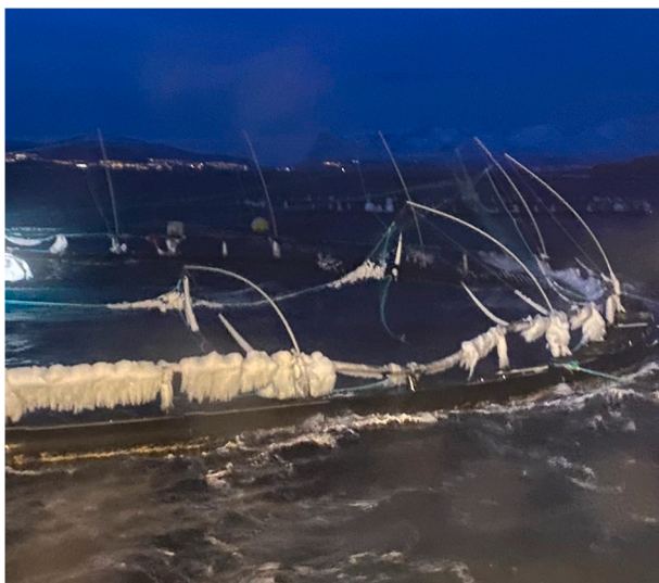
Fig. 24. Damage in a fish cage due to ice accretion in Northern Norway (Picture: Alexander Boiko).
