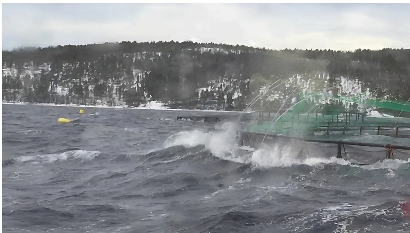
Fig. 30. Illustrating the spray trajectory resulting from collisions between waves and the cage structure during higher wave heights.
