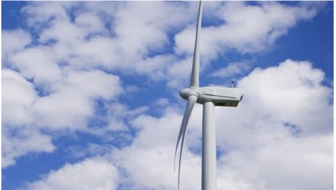
Figure 2. Typical V90 Vestas Nacelle Assembly with Anemometer [63]
