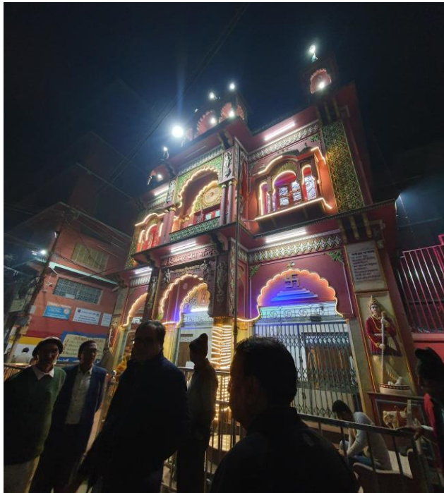
Figure 30: The Digambar Jain Temple in Marwari Patti, Dimapur, Nagaland, was first built in 1947, and has been renovated over the years.
