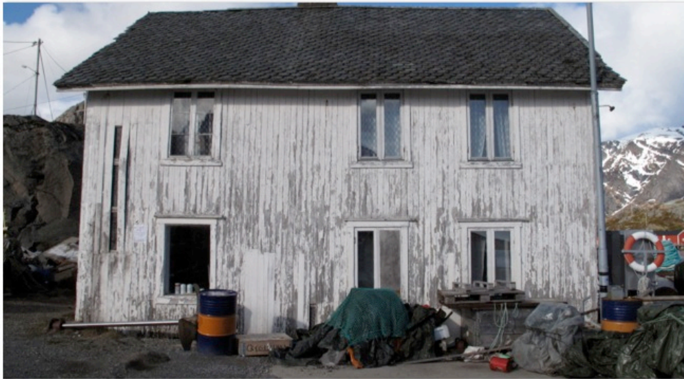
Abandoned house. Sørvågen, Lofoten. Photo: The author
