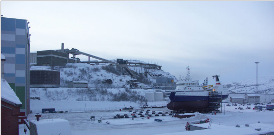
Figure 7.4 The Kimek shipyard in Kirkenes with parts of the Sydvaranger Iron Mine enrichment plant visible on the hill in the background. Photo: Urban Wråkberg
