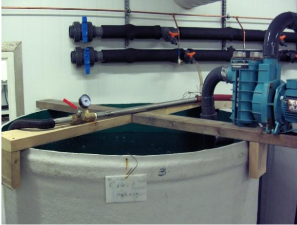
Figure 6. Control setup Marlow pump on scaffold.
