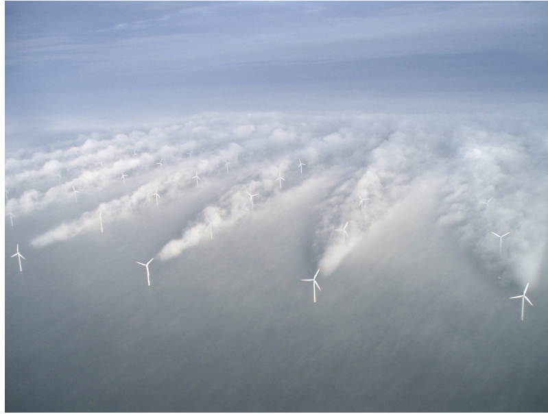
Figure 2.9: Wake effects at the Horns Rev offshore wind farm in Denmark. (Steiness, 2013)
