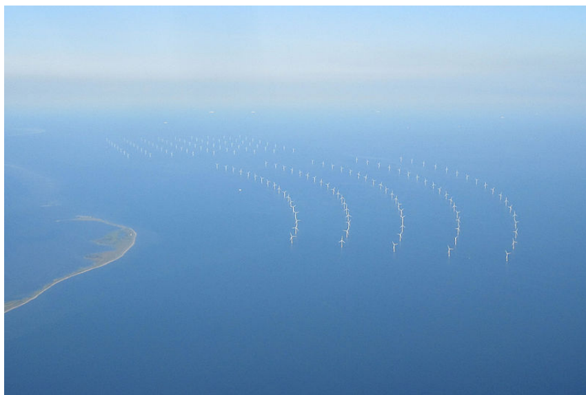
Figure 4.5: The Rødsand II/Nysted offshore wind farms in Denmark.
