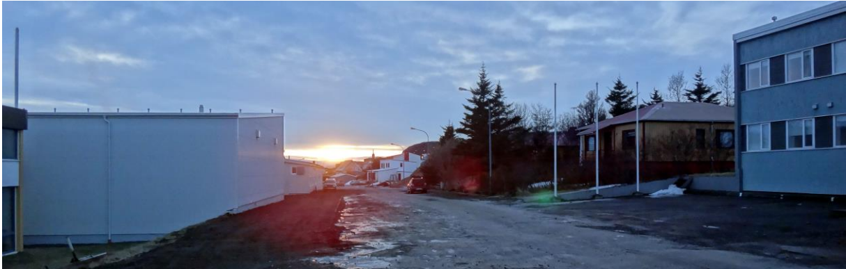
Figure 40. The main street of Vopnafjörður under construction
