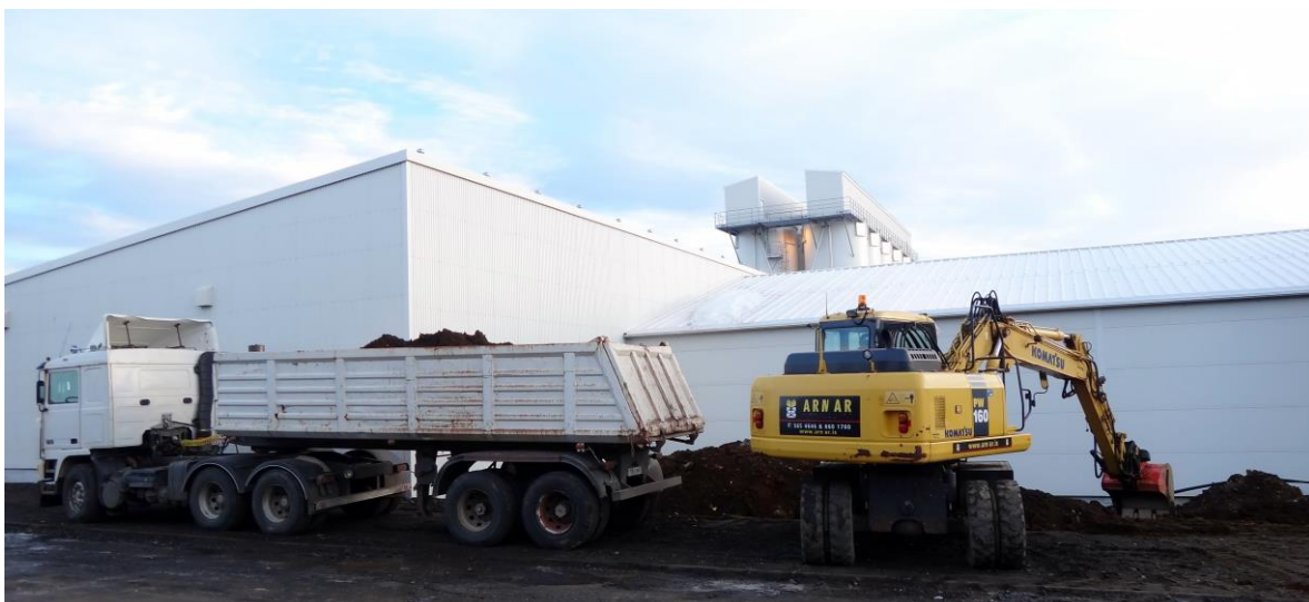
Figure 37. Water pipe installation to HB Grandi facilities (Arnarsson, 2013)
