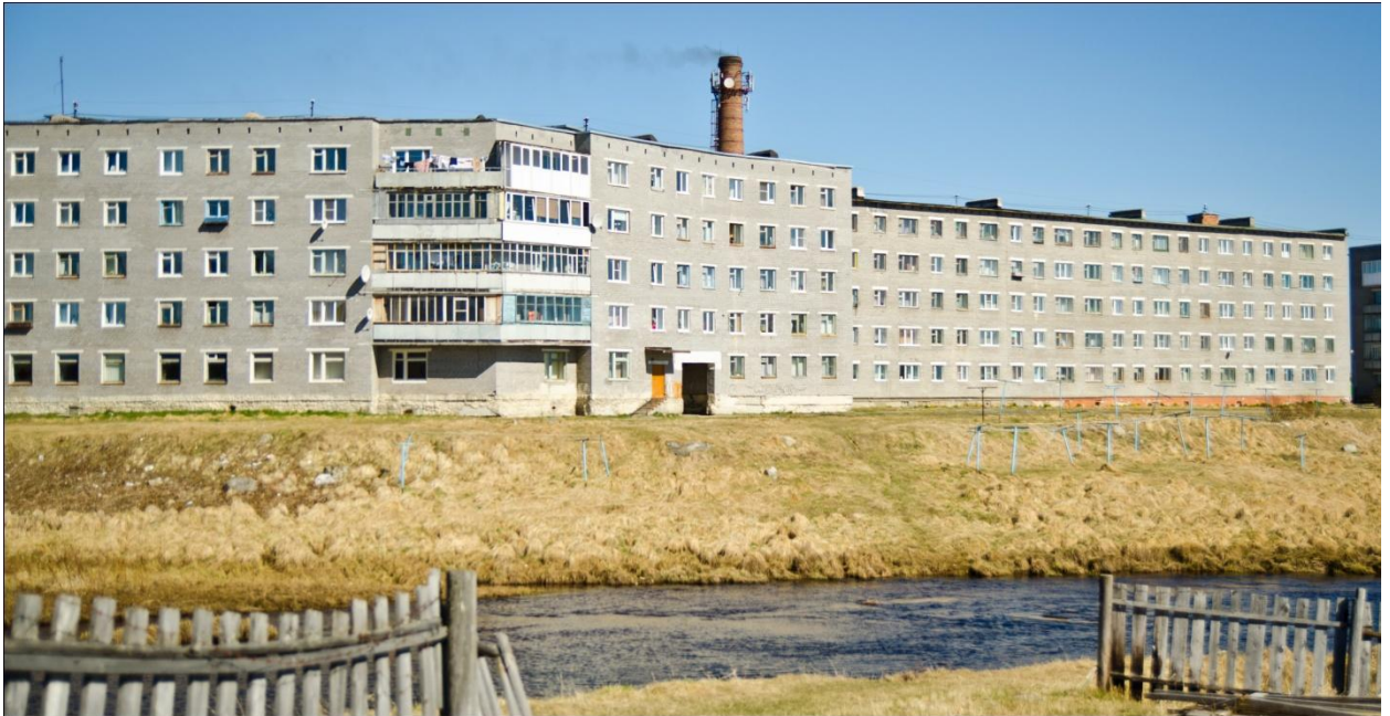
Photo 4: This block of apartments was built especially for the Sami people relocated from Voronye settlement. Beyond the block one can see the pipe of Lovozero boiling station.
