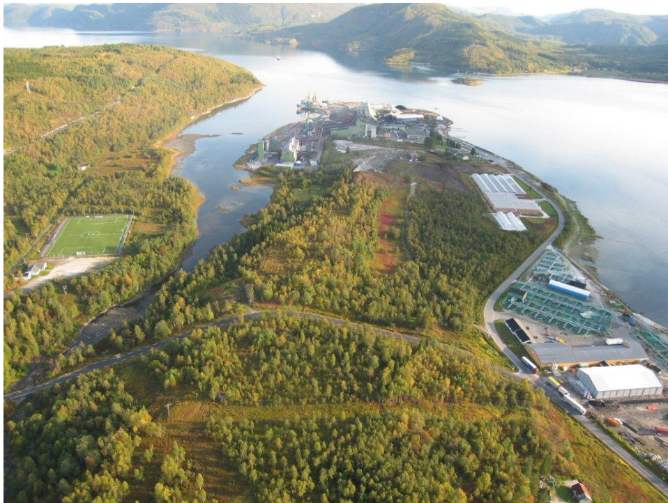
Figure 1.1: Overview of Elkem Salten verk [16]
