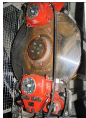
Figure 16 – Conveyor brake
