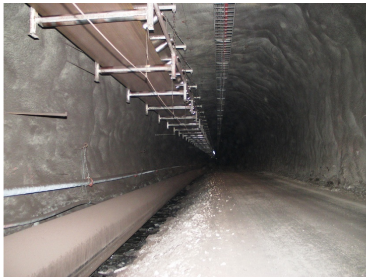
Figure 15 – Mine adit, with the conveyor on top left
