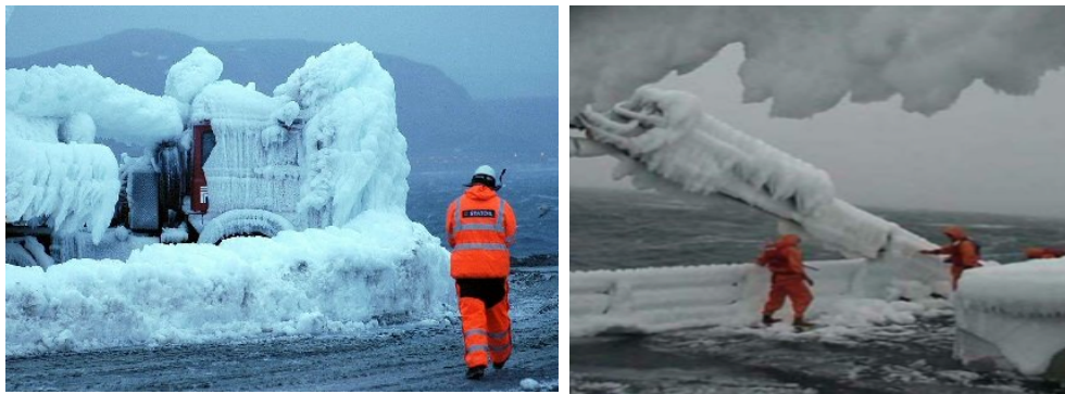
Figure 8: Icing on Snøhvit LNG production facility (Meteorologisk, 2005)
