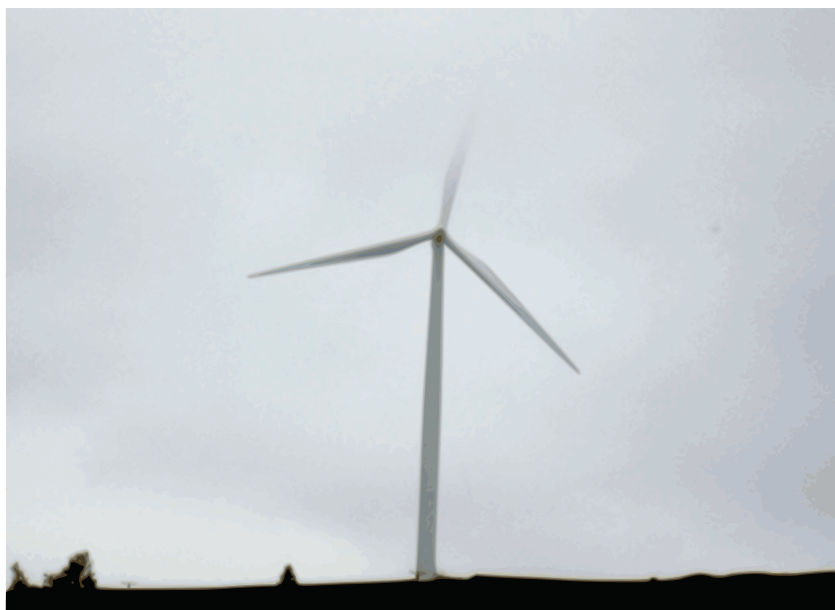
Figure 1.6: Turbine in partial fog, illustrating that the blade tips can extend into a cloud while the nacelle is below the cloud base.
