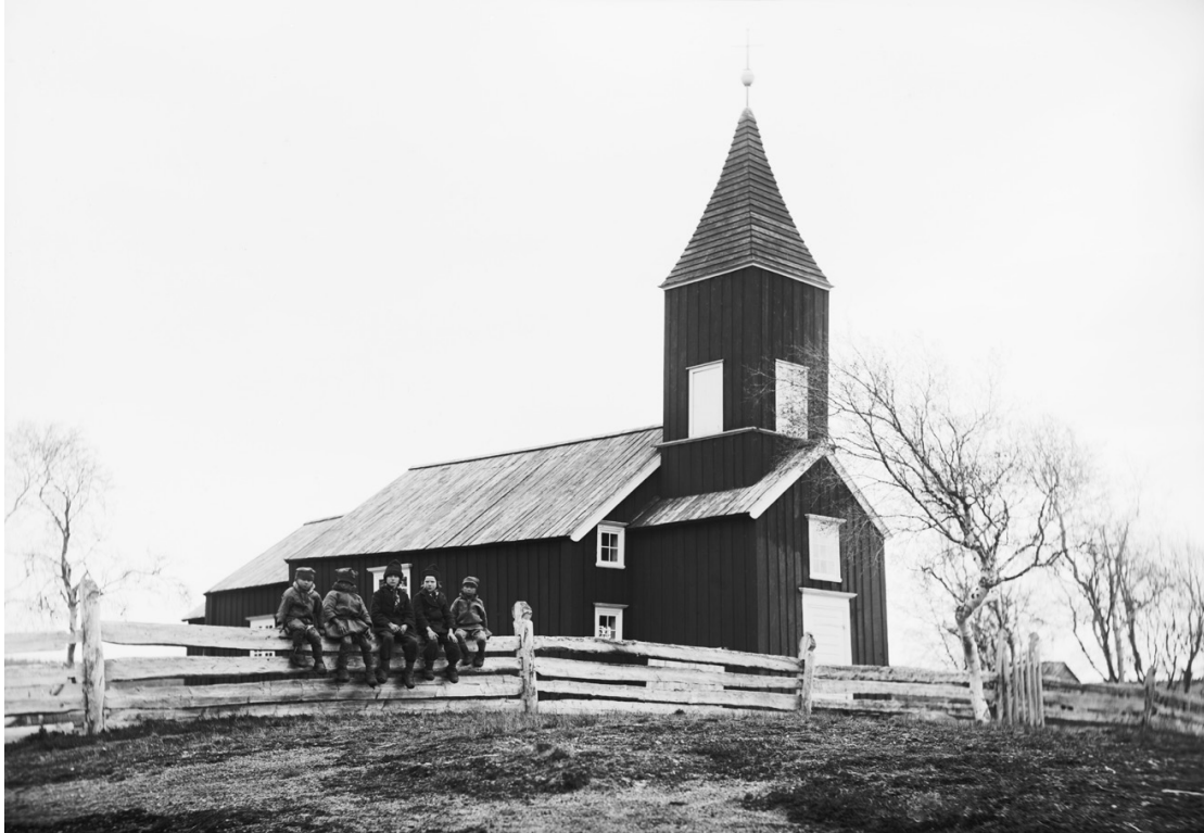
Figure 4 St. Carl, Guovdageaidnu/Kautokeino old church, built 1703. Photo: Sophus Tromholt 1882/83, University of Bergen.
